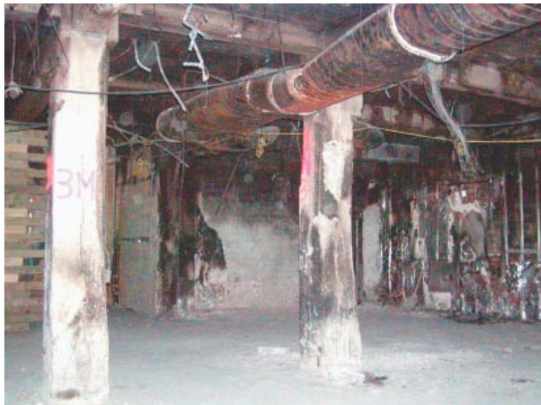
Figure 6.9 First-story columns 3M and 3N
