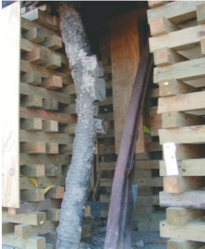
Figure 5.21 Column with triple curvature
