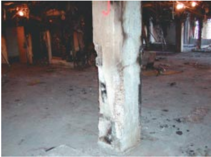
Figure 6.11 First-story column 7J
