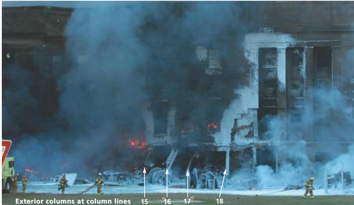
Figure 3.9 Southern portion of impact area before collapse
