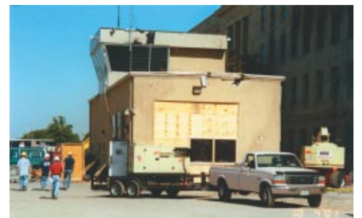
Figure 5.13 Damage to fire station
