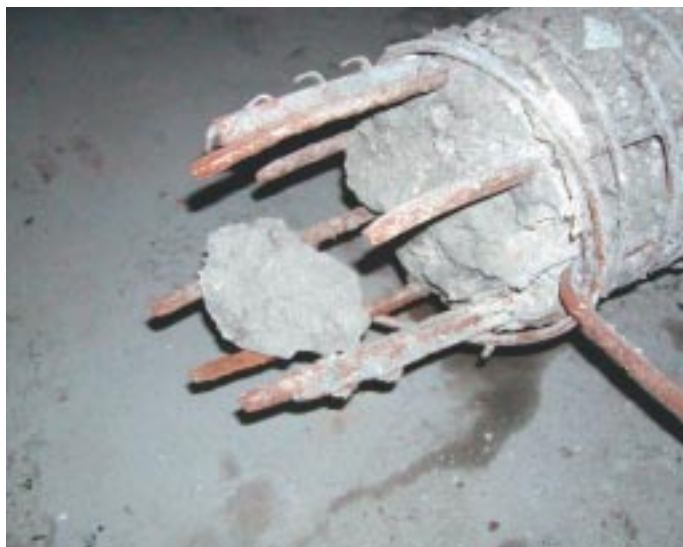
Figure 7.5b Ends of fractured reinforcing bars showing necking
