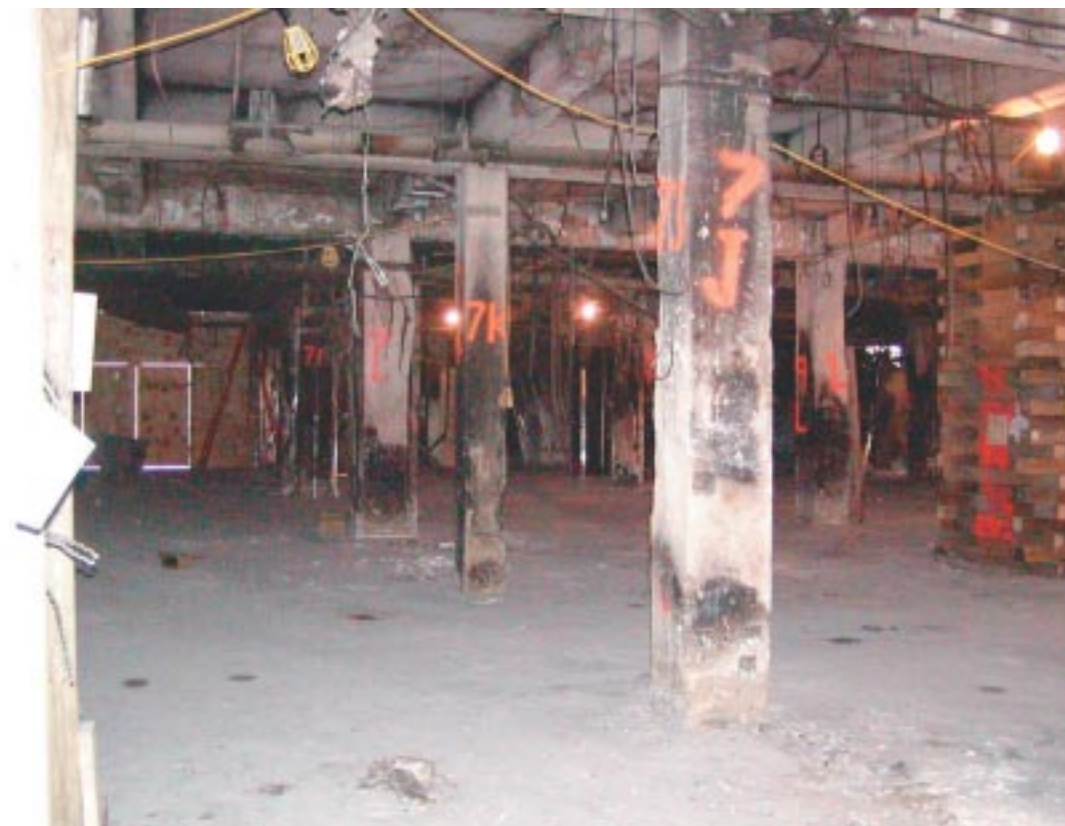
Figure 6.10 First-story columns 7J, 7K, and 7L
