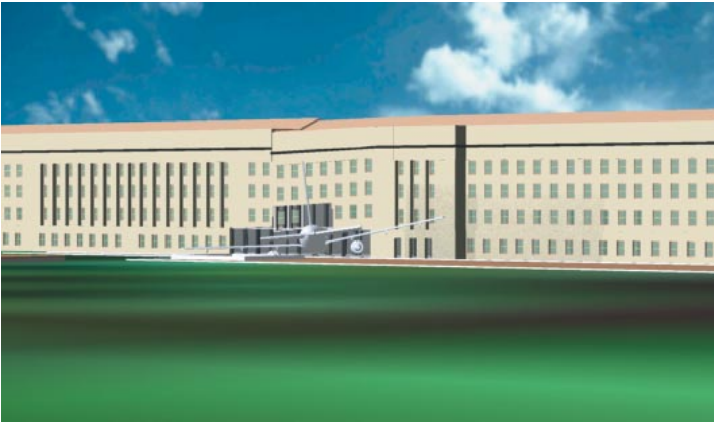
Figure 6.1 Aircraft aligned with damage on west facade
