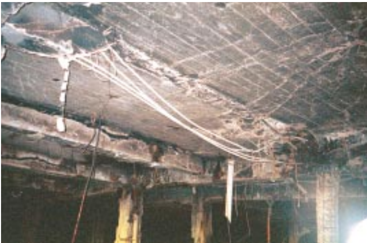
Figure 6.13 Concrete stripped from second-floor beam at grid 9 between grids A and B; extensive cracking in slab
