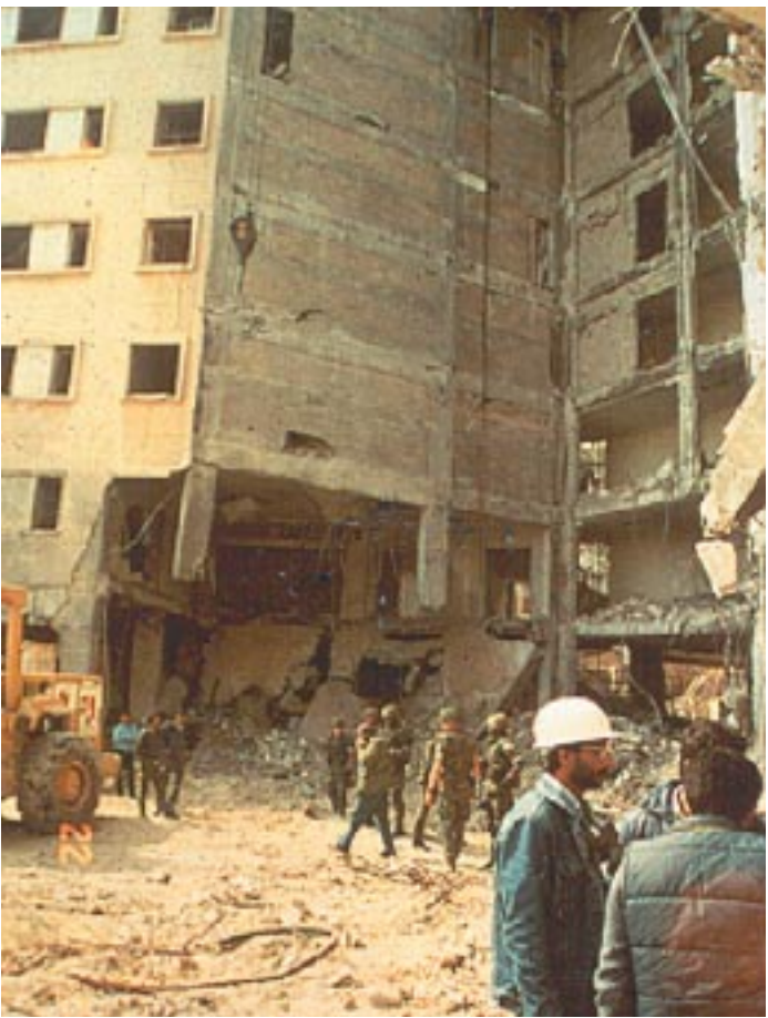
Figure 7.7 Reinforced-concrete frame with masonry filler walls acting as a vertical diaphragm to compensate for column loss
