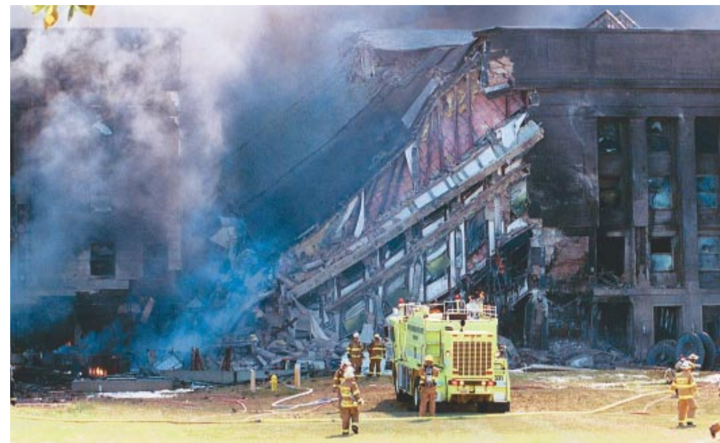
Figure 3.12 Ring E after collapse
