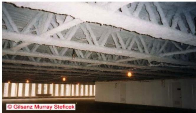
Figure 1–8. Photograph of insulated WTC trusses.
